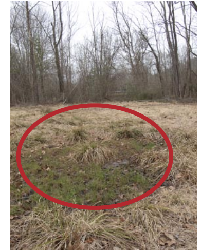
Bog-like conditions (pumping station beyond)
